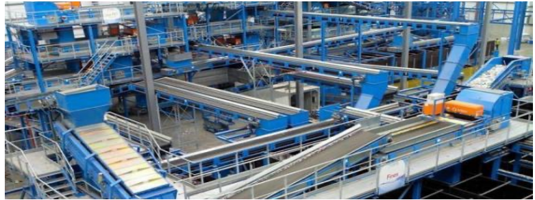
Conveyors – Incremental Encoder used to track speed of conveyor
